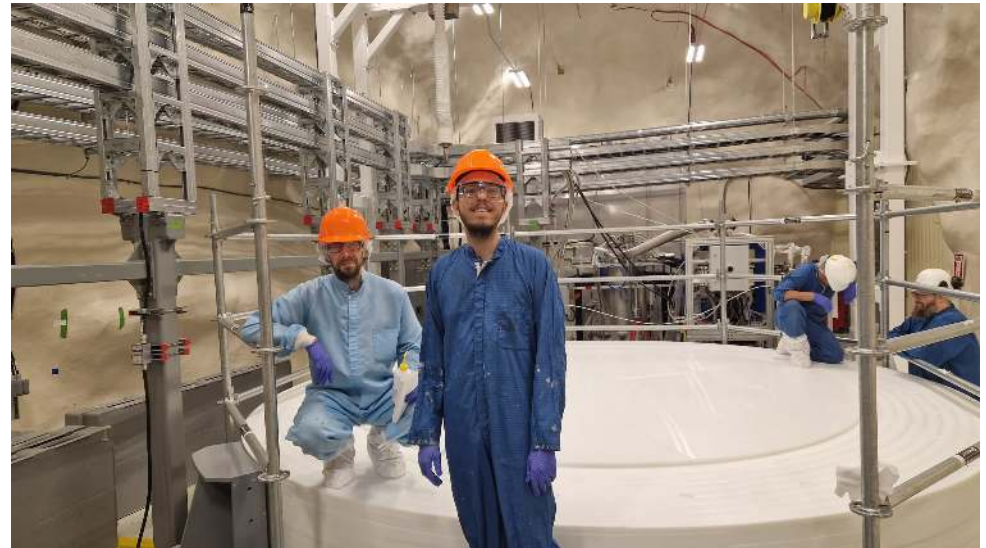
Elías López-Asamar y David Alonso during base shielding installation (May 2023)
